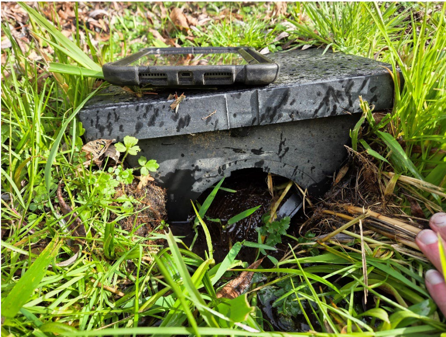
Photo 14. Piped Channel outlets into vegetated slope above bulkhead wall along Lake Washington shoreline.
