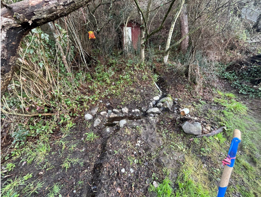
Photo 9. View of the pumphouse overflow channel.
